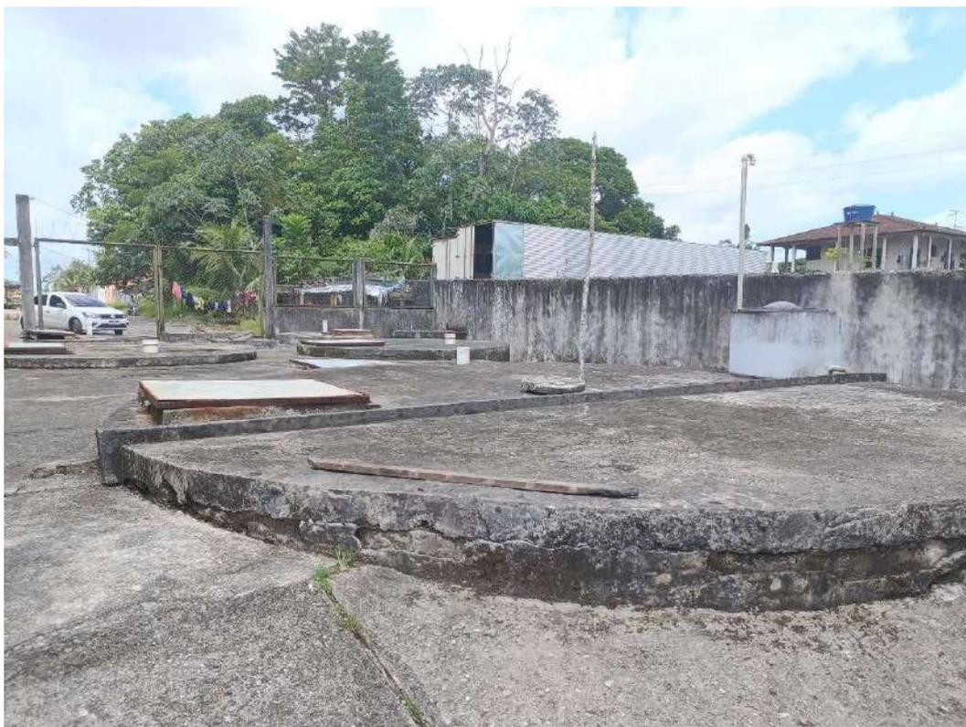
*Figura 279. BEL102-ETE Maracá, laje superior do reator UASB.*
