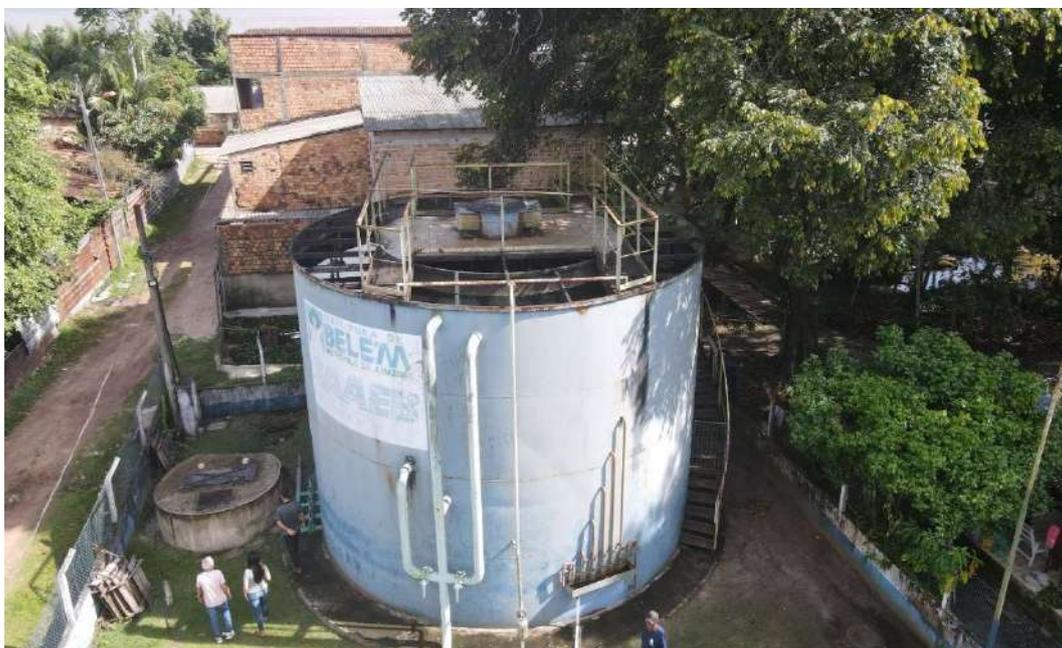
*Figura 298. BEL051-ETE Outeiro, reator UASB compacto.*
