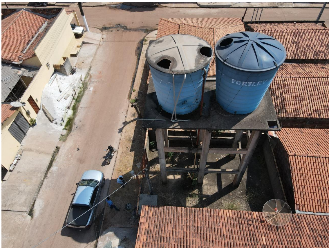
Figura 29. ULI05-REL1 e ULI05-REL2: vista geral.
