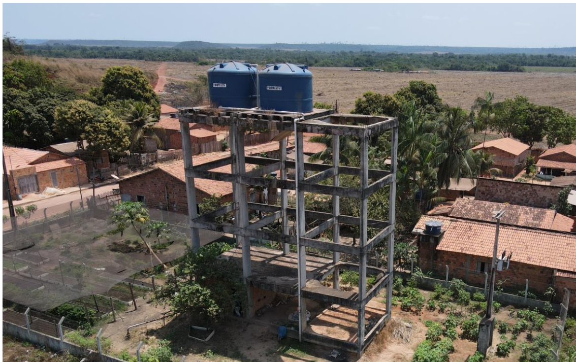
Figura 42. ULI18-REL1 e ULI18-REL2: vista geral.
