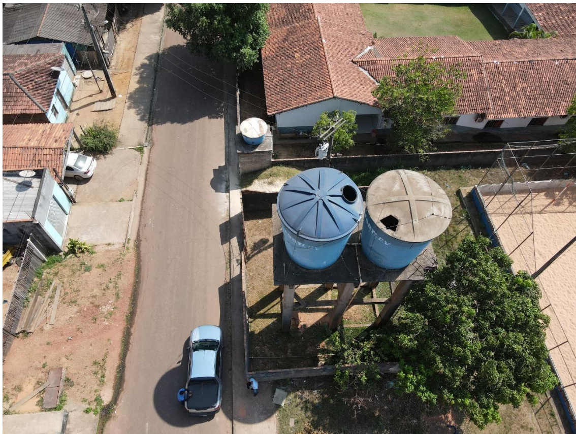
Figura 27. ULI03-REL1 e ULI03-REL2: vista geral.
