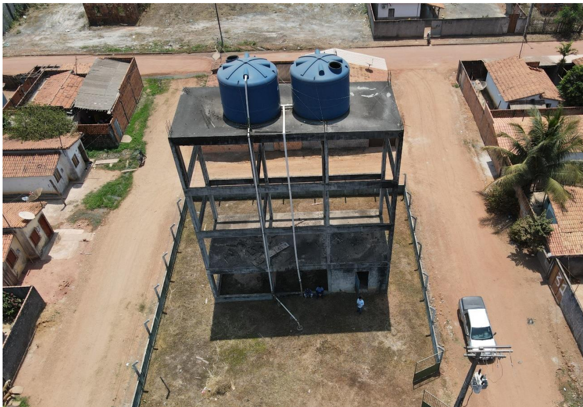
Figura 43. ULI19-REL1 e ULI19-REL2: vista geral.
