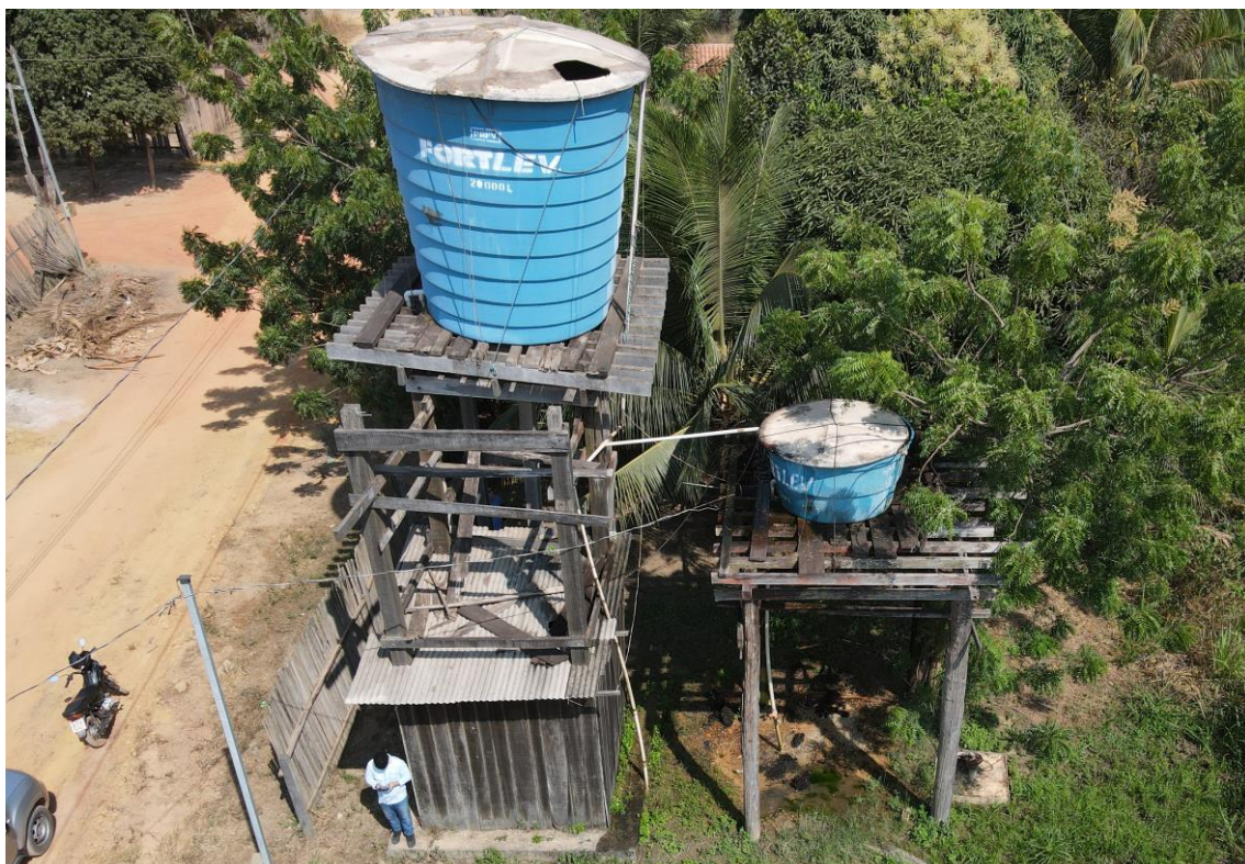
Figura 31. ULI07-REL1 e ULI07-REL2: vista geral.
